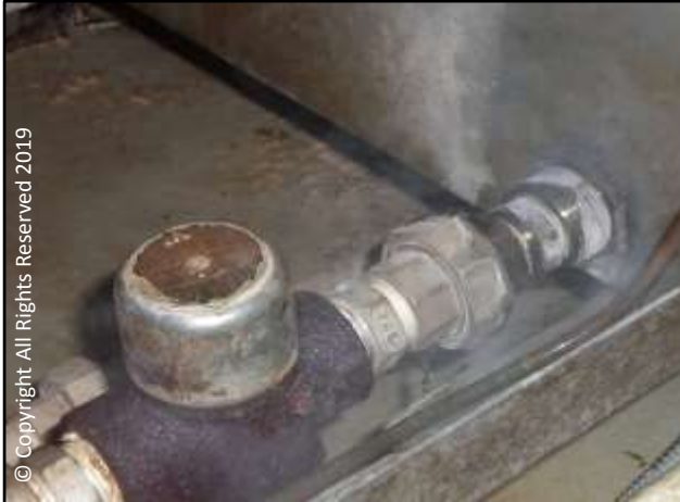
Steam condensate leak flashing to steam, wasting energy and water
